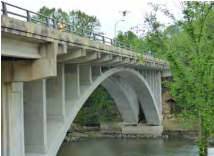
UAV Bridge Inspection Demo Project by MN DOT
