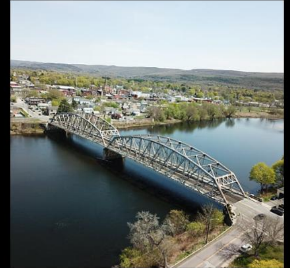
State Route 6 over Delaware River
