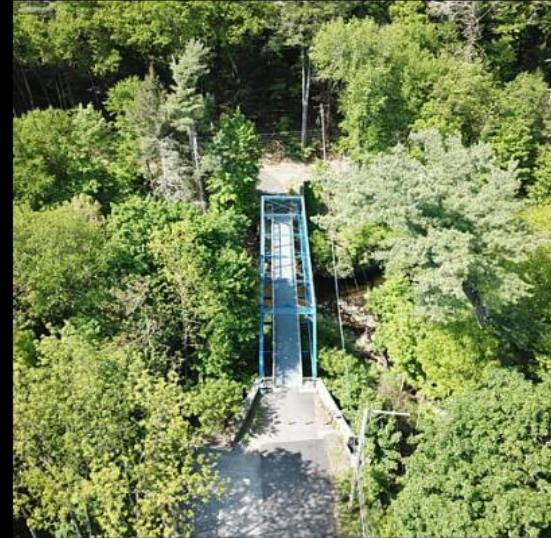
Mott St Bridge
