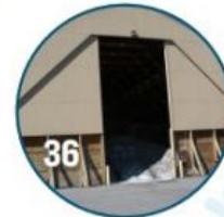
Salt Storage Facilities
