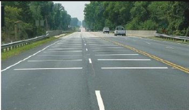
THERMOPLASTIC RUMBLE STRIPS
